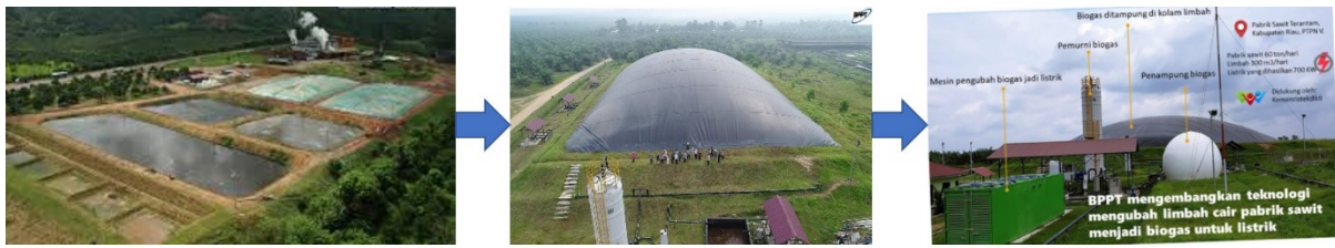
Figure 25 Schematic Illustration of POME Conversion to Biogas for Electricity Production 26
